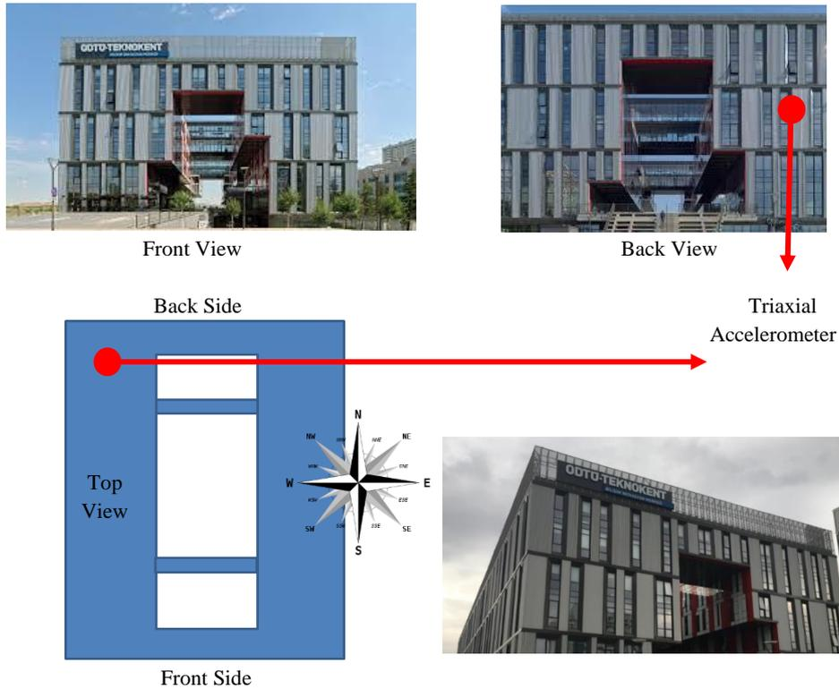
**Fig. 7.** The five-story building monitored with a single triaxial accelerometer and the sensor location
