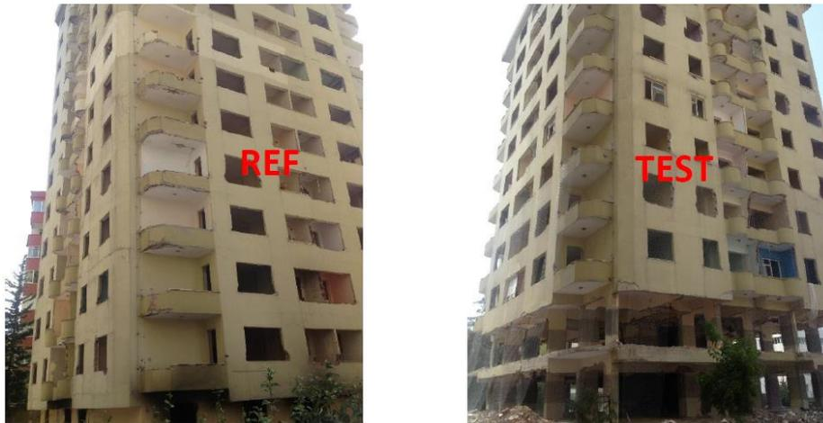
**Fig. 2.** Left: Undamaged – selected as the reference Right: Controllably Damaged – selected to observe the shift in the natural frequency
