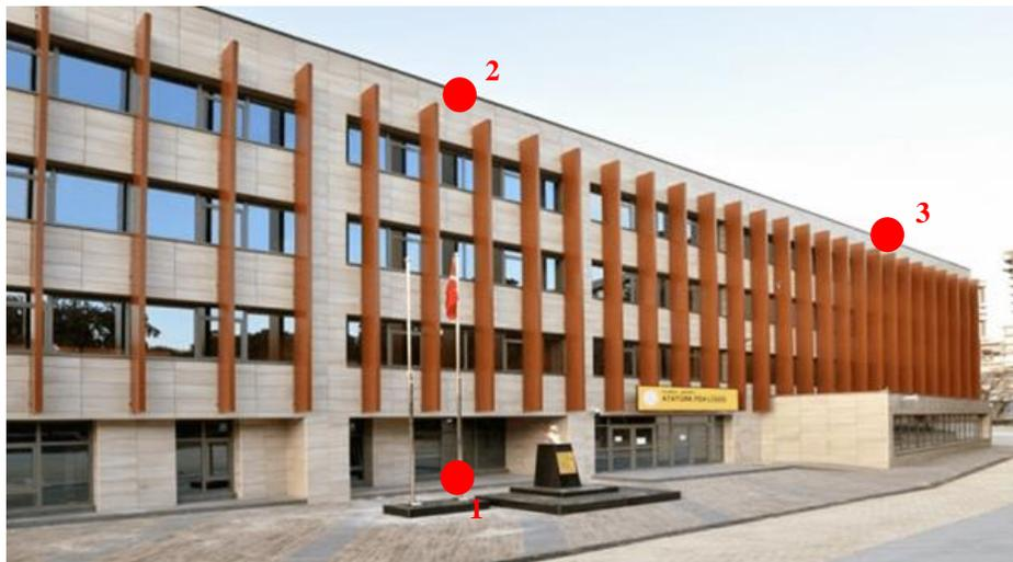
Fig. 9. The three-story school building and the triaxial accelerometer locations
